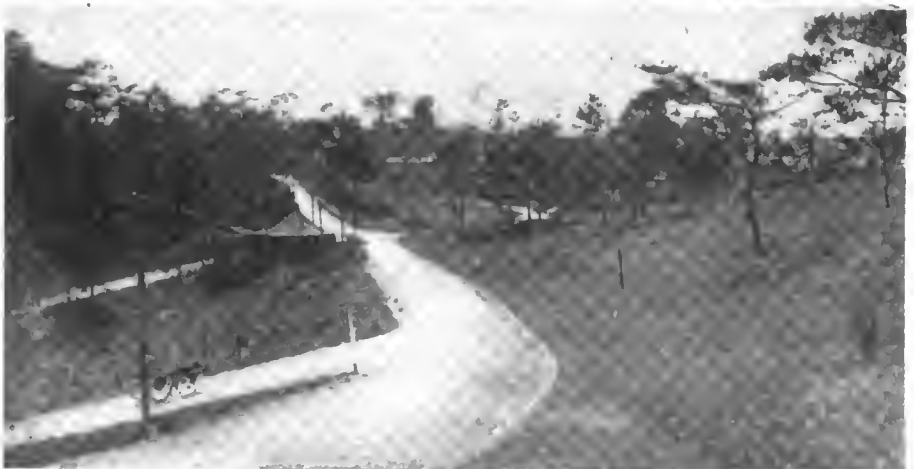
Above is a typical scene on the 115-mile section of the Manila South Road to Atimonan. It is all first class macadam and passes for miles through stately coconut groves. Note the Peerless truck
